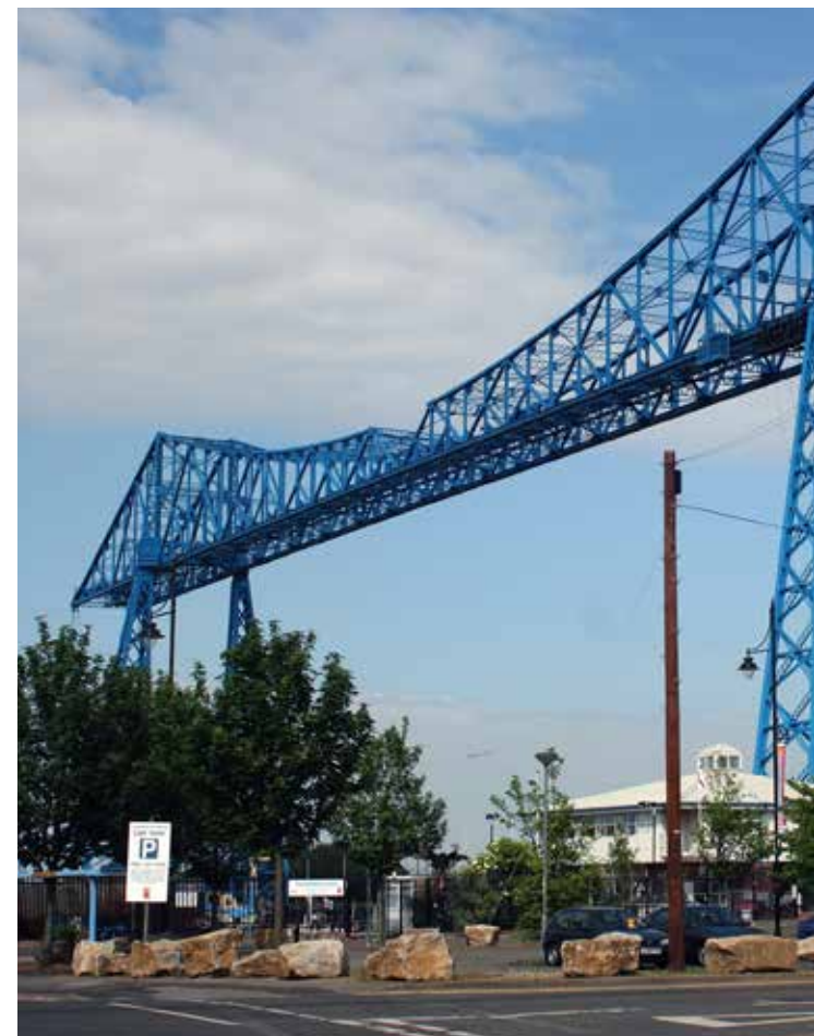
Tees Transporter Bridge
